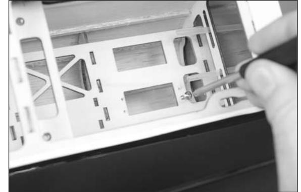
□□ 7. Apply 2–3 drops of thin CA in each hole to harden the surrounding wood. This will help prevent the screws from vibrating loose.
